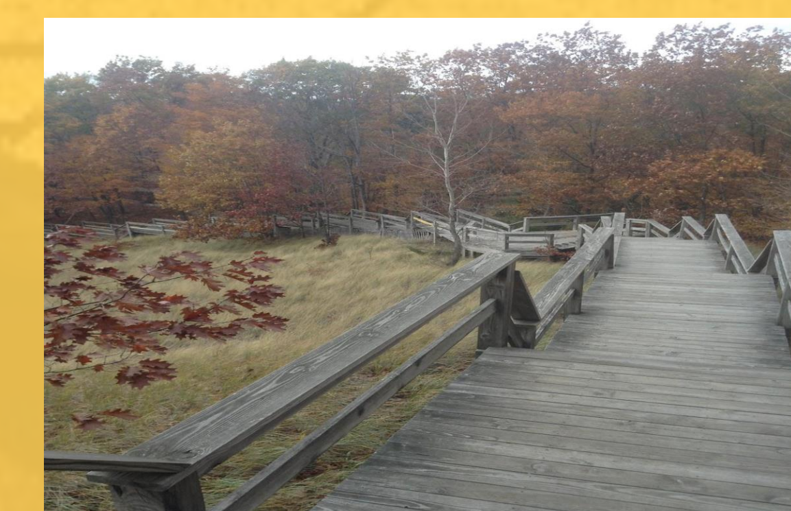
Figure #4: Photo of Dune Climb Boardwalk. This picture shows the study area for this project. It can be noted the weathered look of the majority of the boardwalk. A noticeable gap in the railings can also be seen, big enough to allow someone to pass through.
