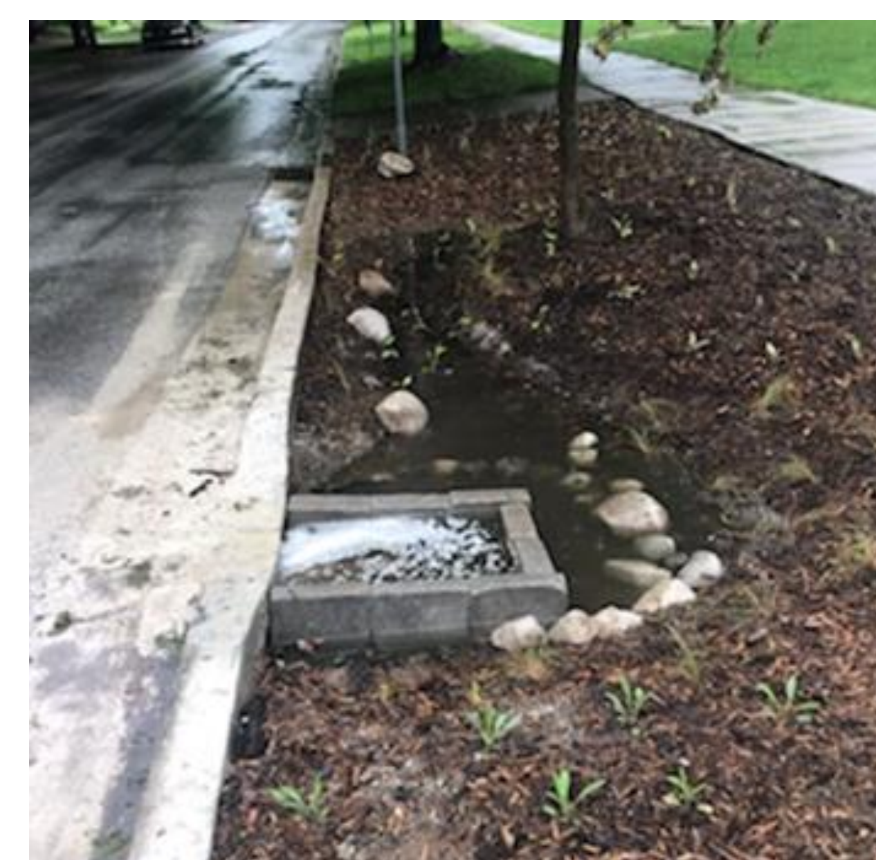
Fig. 3: A sediment trap in a rain garden filling with water, and depositing sediment into the trap that would have ultimately ended up in Plaster Creek.
