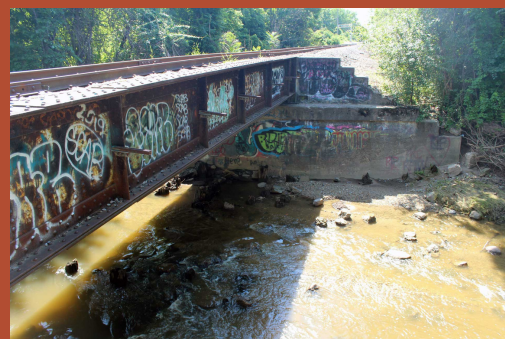
Railroad overpass downstream
